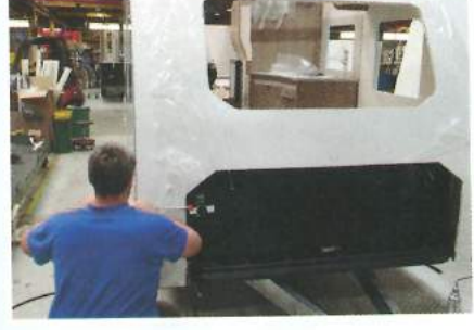
6 Composite wall panels are added and glued and screwed to the floor, then the front and rear panels. Most of the internal structure is already in place. The caravan is now beginning to take shape.
