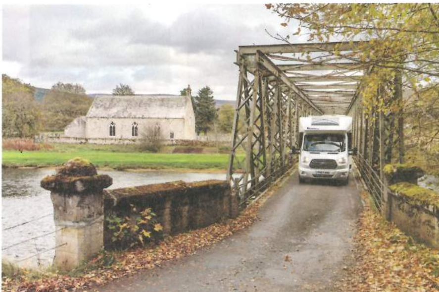
At Cromdale you can cross the steel bridge and, in season, watch the leaping salmon
